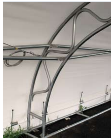
Big Top's arch-style hangar has welded trusses made of S-bend tubing. It's anchored by rods and plates driven into the ground, top.
